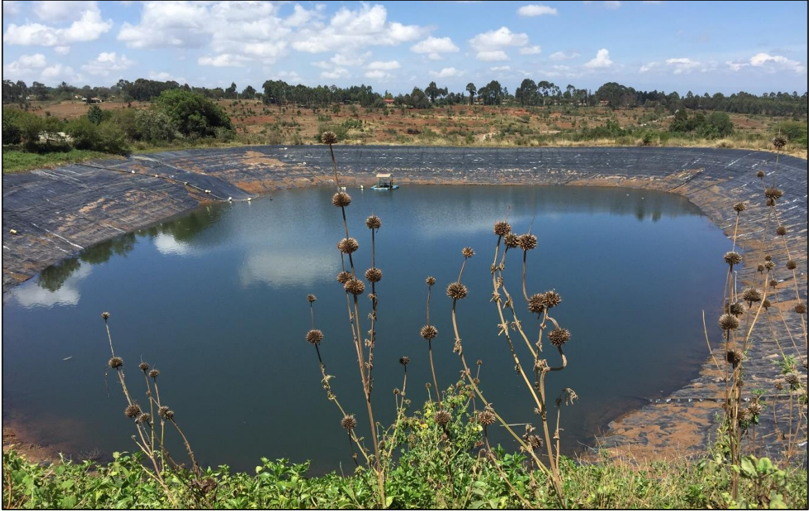
Figure 8: One of several water storage reservoirs (~50,000 m 3 capacity) inside a commercial flower farm in MKWR during the dry season
